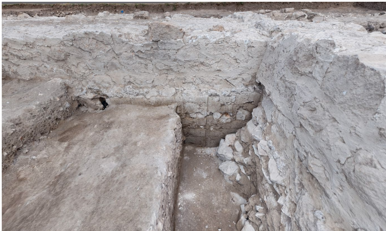
Fig. 10: Ostia antica, Constantinian basilica. Southern side of the foundation of the northern nave wall, view from the south: in the lower portion a refined cast foundation with moulding imprints, above the upper masonry part of the foundation; to the bottom right the deeper, rougher cast foundation of the east wall, while the upper part of the foundation was built in conjunction with the foundation of the northern nave wall
