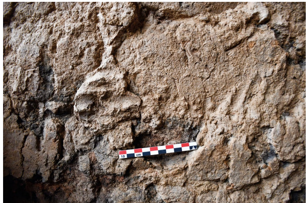
Fig. 29: Close-up photograph of one of the renderings documented in the north corridor of the courtyard of Casas del Turuñuelo, showing the detail of the finger imprints resulting from applying the mortar directly by hand.
