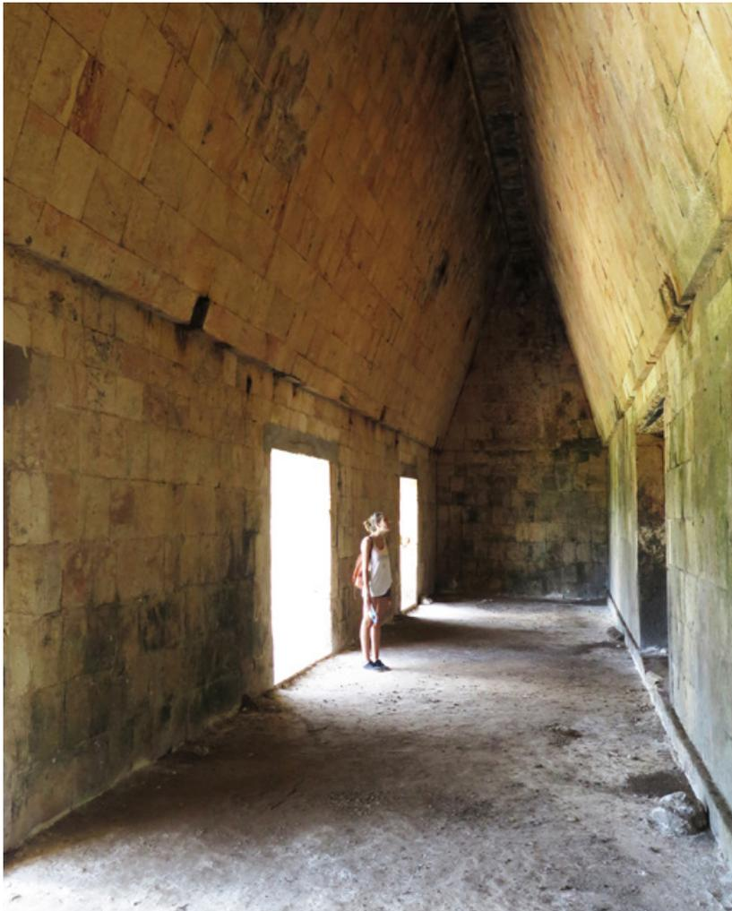
Fig. 16: Vaulted room of the House of the Governor in Uxmal
