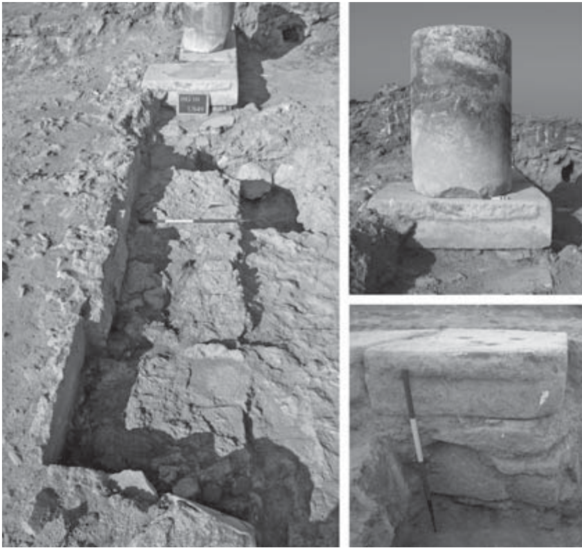
Fig. 36 Hierapolis, Gymnasium, the Byzantine foundations of the portico made of blocks of varying dimensions, reused materials and lay- ers of bricks
