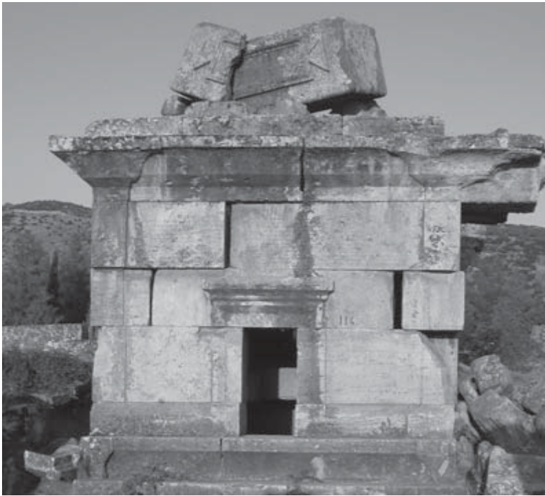
Fig. 2 Hierapolis, North Necropolis. The effects of disastrous earthquakes are visible on the tomb n. 114
