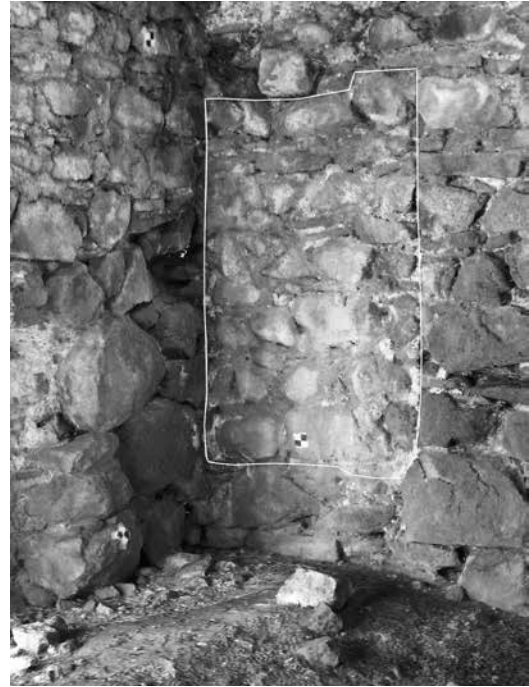
Fig. 10. b Blocked Wall Opening(?) in Room S5
