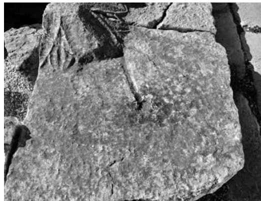
Fig. 5 Northwest corner of the canopy roof
