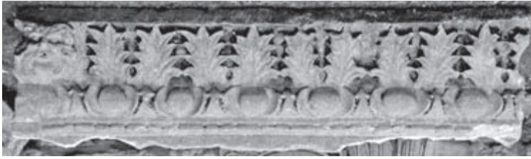
Fig. 145 Inv. 6291, revetment architrave; unearthed together with inv. 6305 as above Fig. 142 ; H 38 L 160 W 2 (bottom) – 22 (top)
