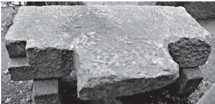
Fig. 72 Inv. 60.54 as above Fig. 70, backside with corner joints and a protruding centrepiece (L 81 W 30)
