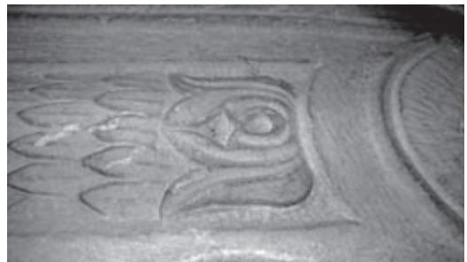
Fig. 44 Inv. 08.36 as above Fig. 41 , end of the soffit on the underside
