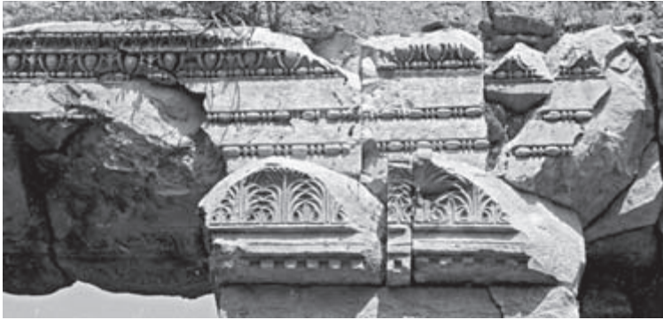
Fig. 122 Antalya, Cumanin Mosque, ancient entablature parts reworked in the sixth century; the cornice is re-used as pier capital and thus placed under rather than above the architrave
