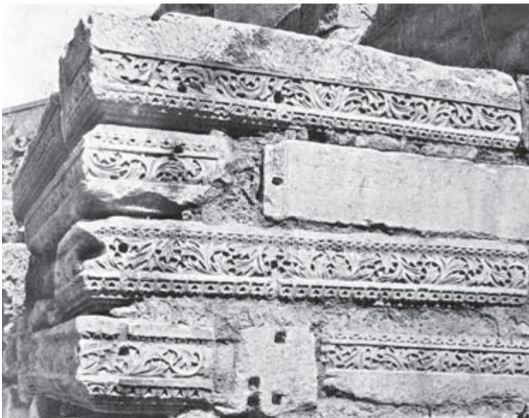
Fig. 90 Boukoleon Gate, re-used architrave; six or more blocks, at least four of which form corners, each with a long and continuous side and a short side that, where visible, terminates in a boss
