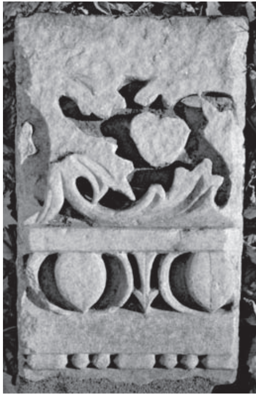
Fig. 82 Inv. 44.30, revetment architrave; from the Koca Mustafa Paşa Mosque (St Andrew in Krisei) in 1931; H (broken) 56 L 33 (bottom) – 36 (top) W 5; broken at the bottom that is covered with cement mortar, and damaged at the top
