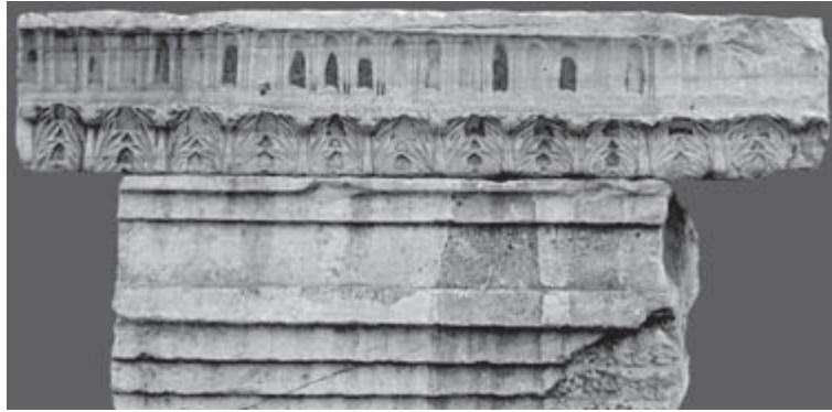
Fig. 23 Arch of Theodosius, architrave with embossed frieze and cornice with a row of soft-pointed acanthus leaves below and fluting above
