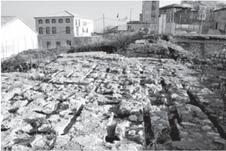
Fig. 25 Grooves of the wooden beams under the floor of the church at ›Anemas Dungeon‹
