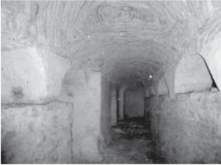
Fig. 4 Parallel walls in the substructure of the North Building
