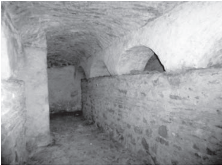
Fig. 5 Interior of the substructure of the North Building
