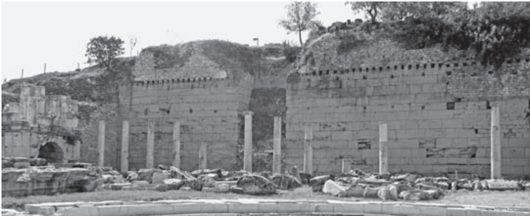
Fig. 1 General view of the South Stoa facing south, with East Gate to left and theater hill retaining wall behind
