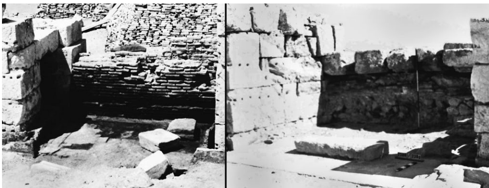
Fig. 74: (left) The north-western recess (in brick). (right) The south-western recess (in opus vittatum ).
