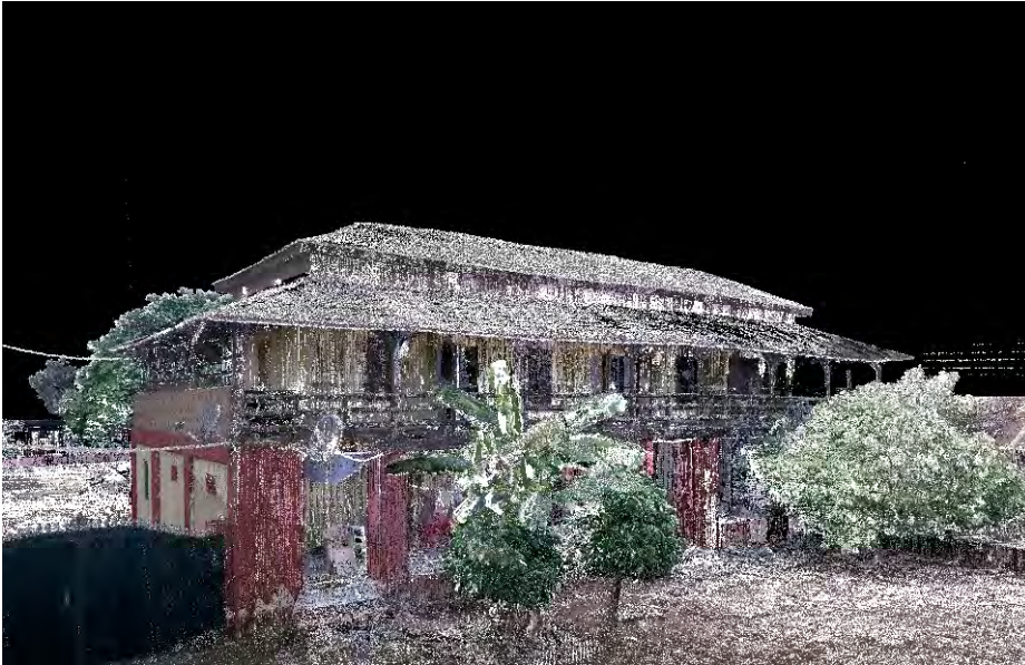
Fig. 3: Kpando, Ghana. Digital 3D model of the Palace of the Paramount Chief incorporating data from laser scanning measurements
