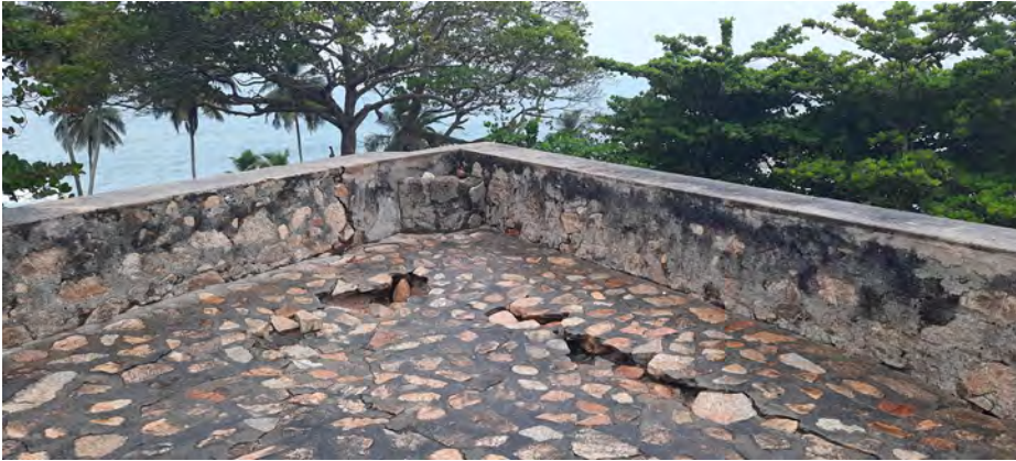
Fig. 10: Princes Town, Ghana. Even though parts of Fort Gross Friedrichsburg seem well preserved, a lack of regular maintenance measures is apparent. Damage to roofs, windows, doors, walking surfaces and water drainage systems is accelerating, leading to structural damage in the buildings and fortifications, such as the western bastion
