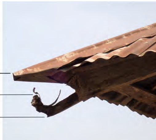
Fig. 9: Kpando-Todzi, Ghana. The rainwater drainage systems on the roofs of all the buildings were also documented. In the case of KT 005, one of the outbuildings of the German administrative station, several phases of repair or reworking were identified
