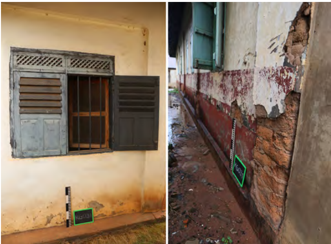
Fig. 7: Kpando, Ghana. House KG 031, for example, shows the elaborate design of the shutters with decorated transom and partial louvers for optimal ventilation (left). While the front side is in very good physical condition and therefore, does not allow any conclusions regarding the building material, fired bricks could be documented on the back side (right)
