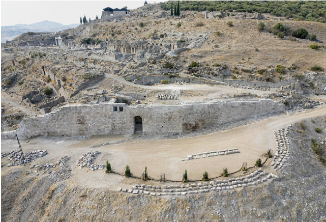
Fig. 8: Monument conservation, Great Gymnasium. The restored east wall after consolidation of the area in front of it
