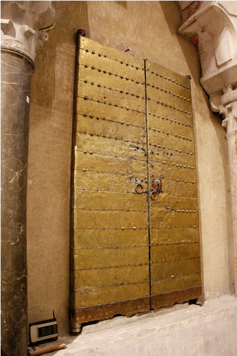
9 Door leaves of the 10 th century covered by brass bands at the Mosque-Cathedral of Córdoba (Spain). (Photo: Alejandro Ugolini Sánchez-Barroso)
