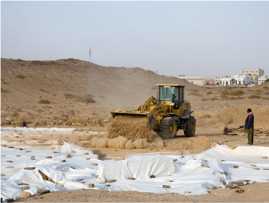
2 Tayma, Saudi Arabia. Examples of conservation and restoration techniques: Backfilling. (Photo: Hausleiter 2018, Fig. 8)
