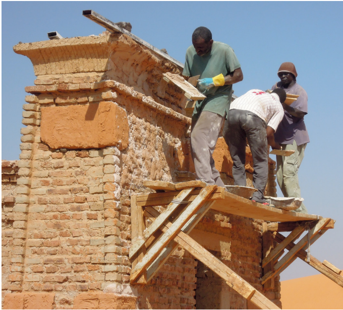
12 Reconstruction work at the chapel of pyramid Beg. S. 10. (Photo: © QMPS, T. Bunk, 2017)
