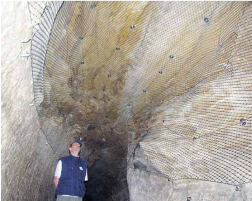
Fig. 19. The wire net with the anchors (Ch. 660)
