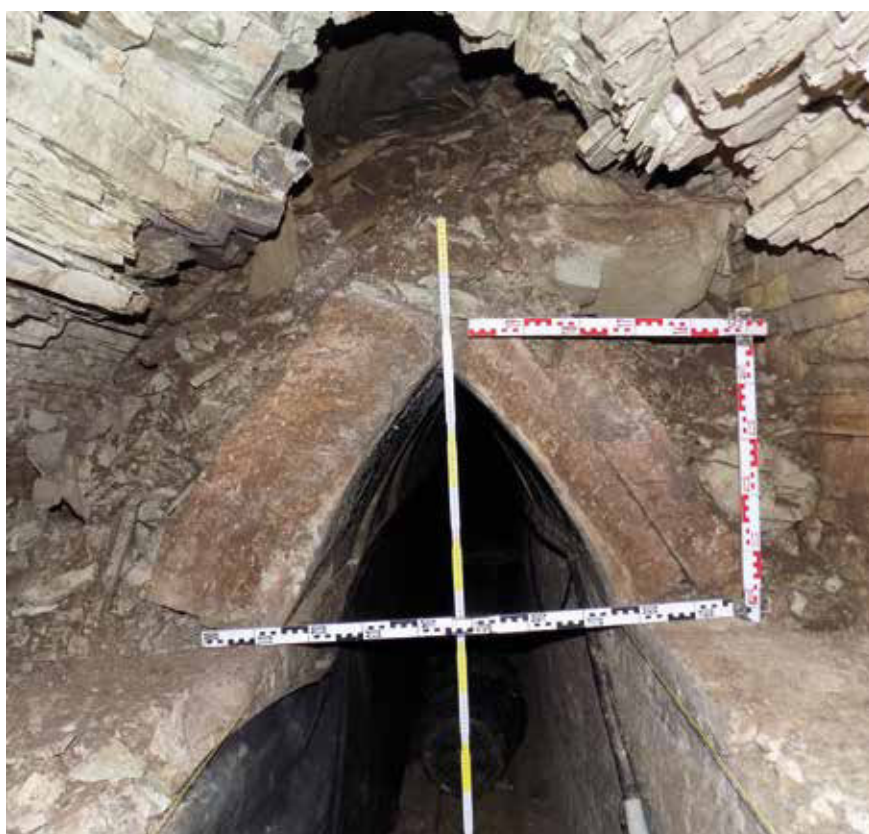
Fig. 22. The dismantling of the slabs of the archaic lining at Ch. 178.6, view from south
