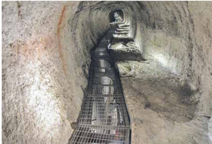
Fig. 24. The tunnel with the steel gratings and the new illumination with LED lights, view from the north (from Ch. 855, before the inscription ΑΡΙΣΤΕΙΛΩ)
