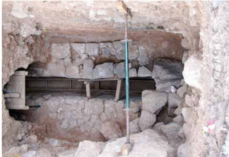
Fig. 23. The excavation near the south portal and the dismantling of the blocks of the roof of the Archaic lining, north on the left
