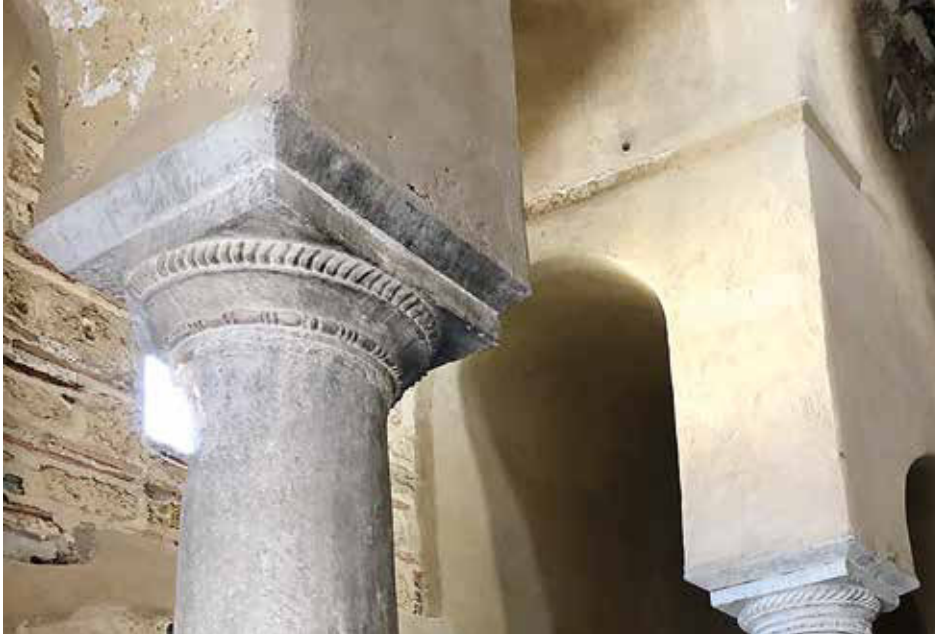
Fig. 32 Metamorphosis tou Soteris, Ionic-Attic bases reused as capitals on the first and second left column
