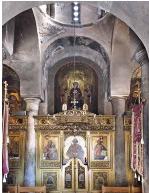
Fig. 43 Agioi Asomatoi, Ionic-Attic base reused as capital on the second left and right columns
