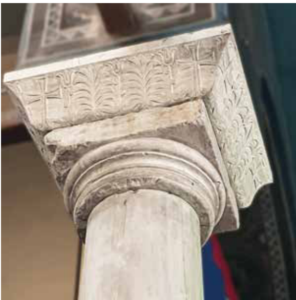
Fig. 47 Sotera Kottakis, Ionic-Attic base reused as capital on the first right column
