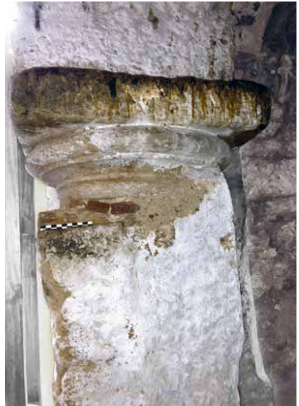
Fig. 33 Metamorphosis tou Soteris, Ionic-Attic base with an upside-down plinth reused as capital
