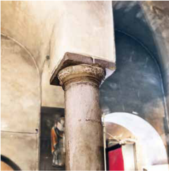
Fig. 42 Agioi Asomatoi, Ionic-Attic base reused as capital on the first left column
