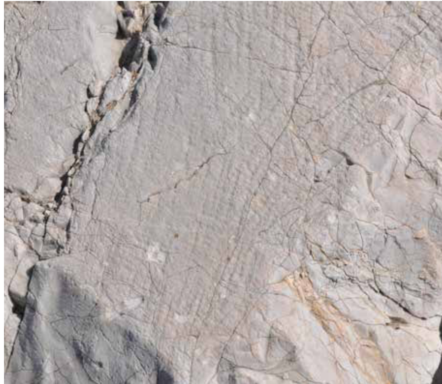
Fig. 3 Dörpfeld foundations, inner blue foundations, detail of claw-tooth chisel marks on block 19
