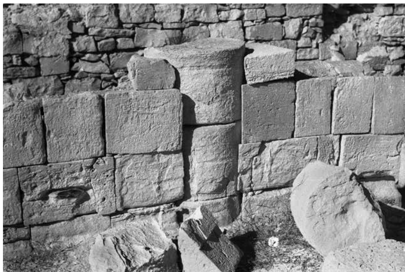
Fig. 22 Rehovot-ba-Negev, Northern Church. An ancient column within a wall that was built in order to protect it from possible future destruction
