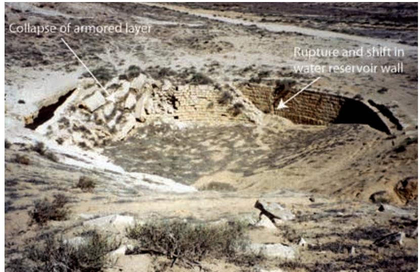
Fig. 18 Rehovot-ba-Negev, seismogenic (?) rupture at the SE wall of the water reservoir. The reservoir was partly cut out of the bedrock and is partly brick-built. Also note the collapse of a significant part of the armored layer which partly covered the reservoir from SW
