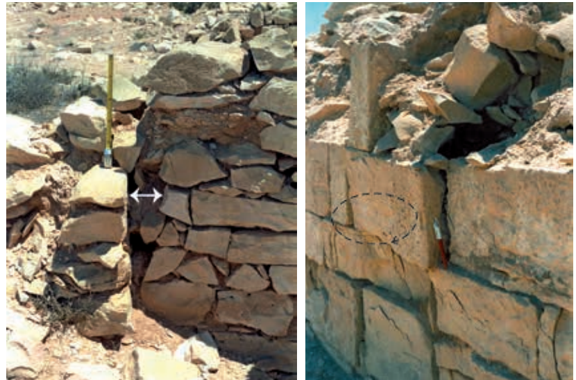
Fig. 16 Clockwise rotation of a stone in an eastern wall (field station 9)
