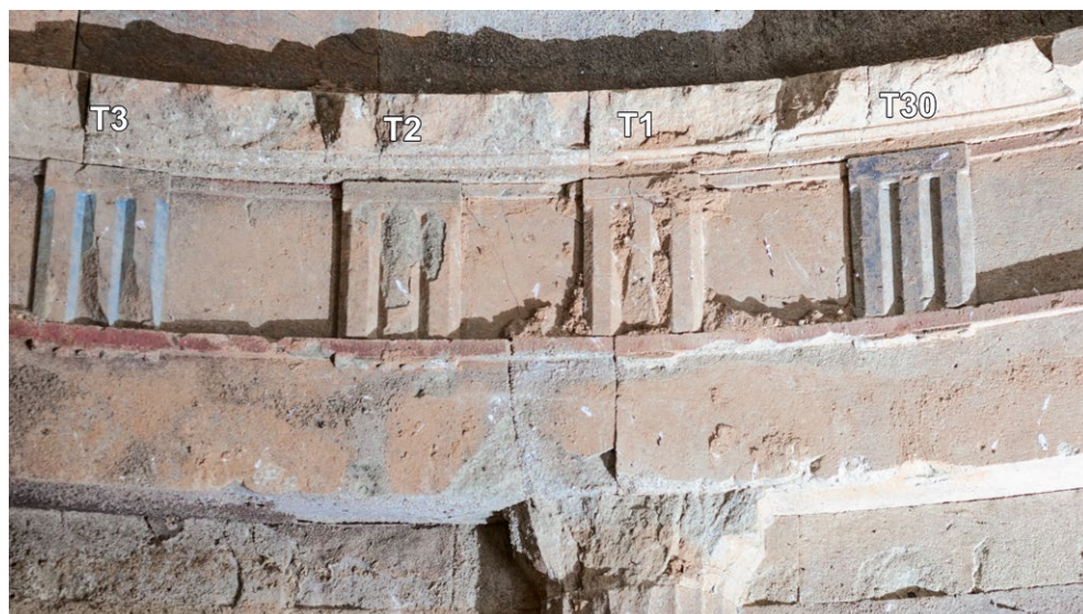
Fig. 100: Starosel. Detail of the entablature above column A, showing an omitted half-regula, and a heavily contracted metope between two unpainted triglyphs
