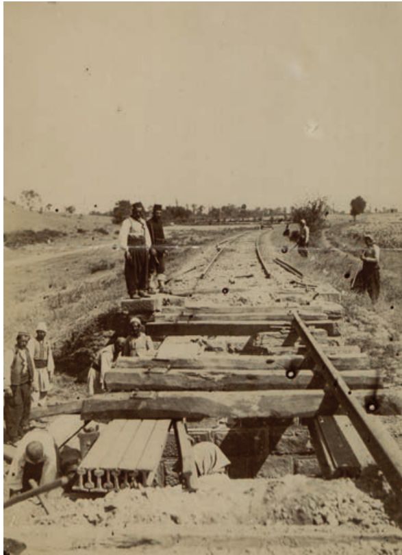
5 Photo of workers building a rail track
