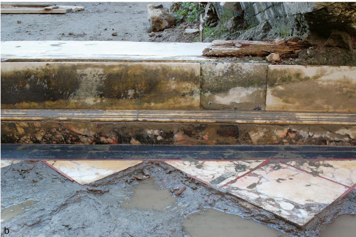
7 a. b) Interior of seaside pavilion (VPSO) from above, with collapsed wall segment in centre. N. B. – opus sectile floor, with wide doorway at top, and base associated with statue of an Amazon at upper left
