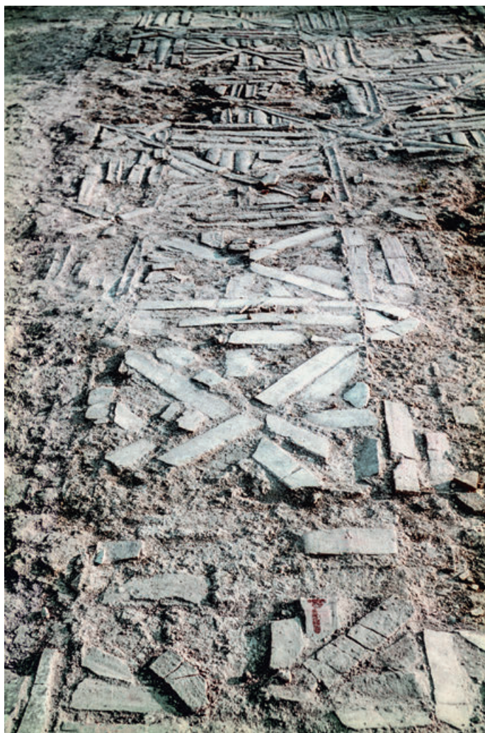
Fig. 15a–c. Gamzigrad, hall 7, detail of the substructure of the cut tile floor (photo by M. Medić, processed by N. Borić, photo documentation of the Institute of Archaeology, Belgrade).
