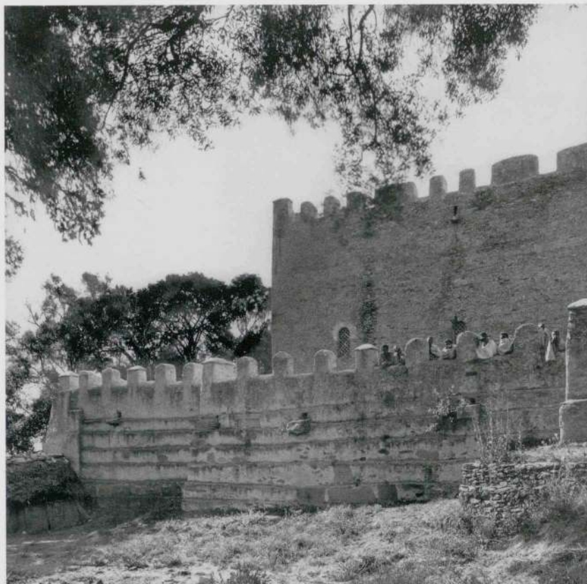
Fig. 7 The north wall of the podium (DAE 2: Abb. 290).
