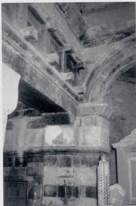
Fig. 21 Zarema Gyorgis, interior of the old church (photo: P. Henze).
