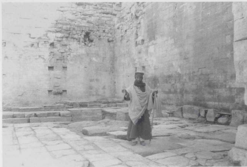
Fig. 5 View of the hypostyle hall after excavation.
