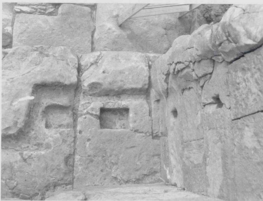
Fig. 14 Some of the grooves visible below the jambs of the entrance, to take a wooden frame for the door.
