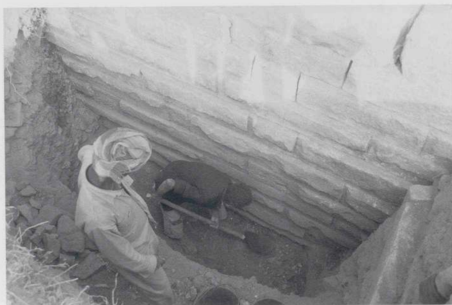
Fig. 12 The foundation courses along the western side of the pronaos.
