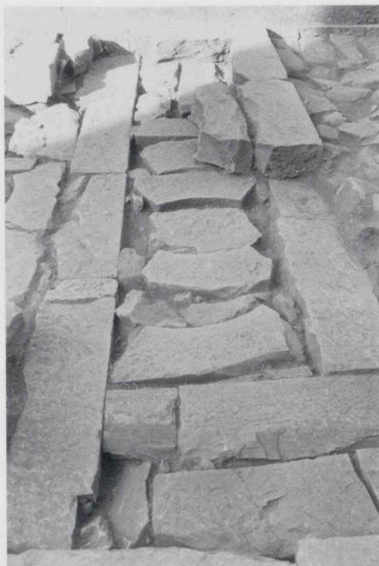
Fig. 8 Fragments of an ancient well-head used in the in-filling in wall M6.
