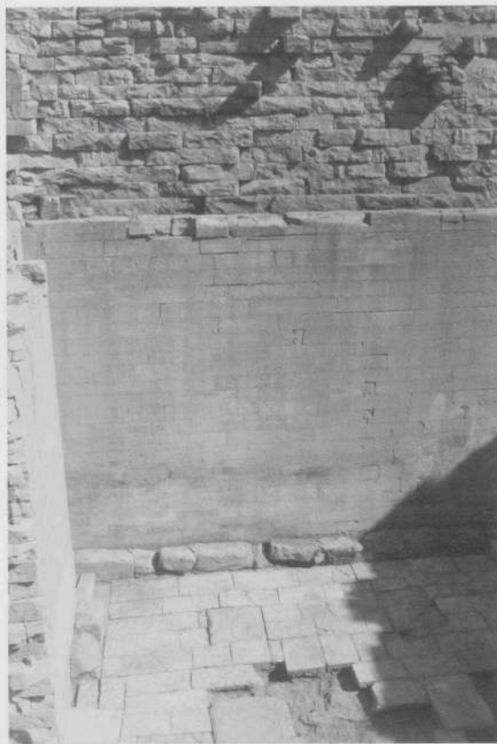
Fig. 3 The ledge running round the interior of the temple at the height of the second storey.
