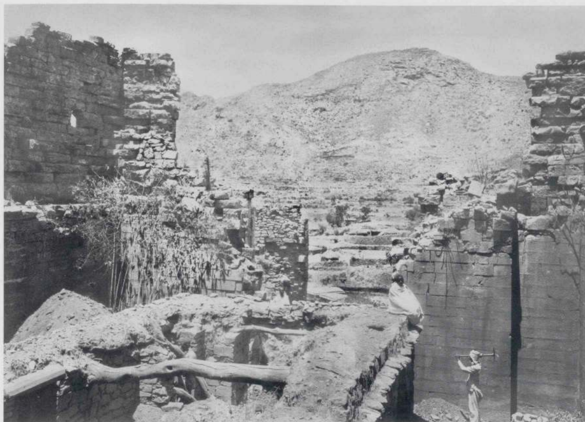
Fig. 10 A previously unpublished DAE photograph by T. von Lüpke (photo DAE 385 = MBA 252.09), showing the interior of the Great Temple at Yeha as seen from the east. In the foreground may be seen the roofless remains of the inner building erected when the Temple was re-used as a Christian church. In the background, beyond the Temple wall, may be discerned part of the western extension built at the same time on the site of the former portico.
