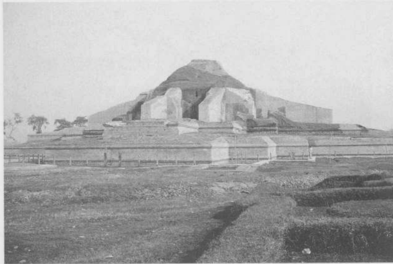
Fig. 4. Pāhārpur's main temple in 2002 (south side), after recent restoration (Breuil/Gill).
